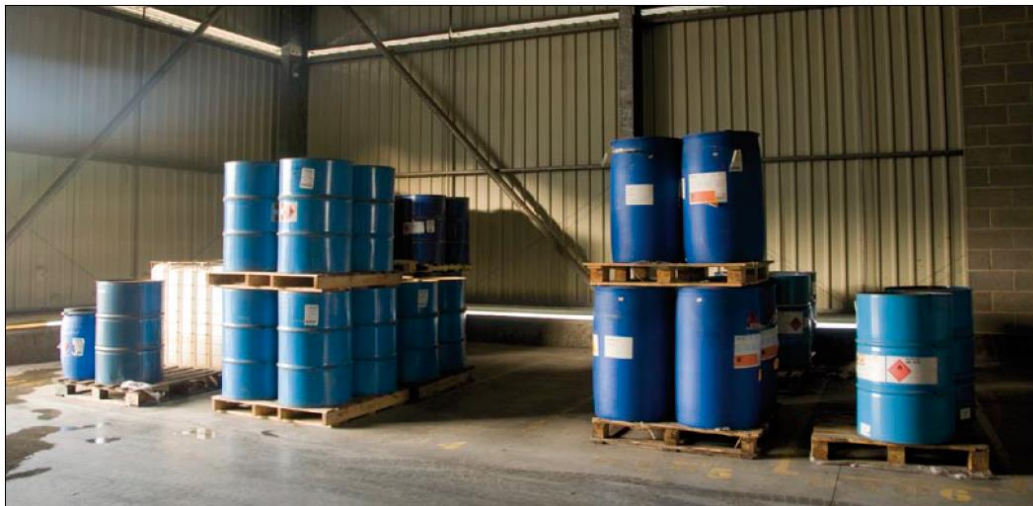
A purpose built, banded chemical drums store
