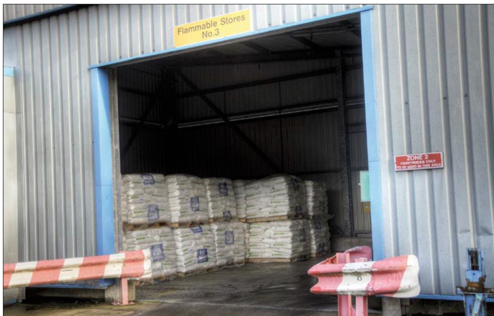
Segregated and bund chemical storage area
